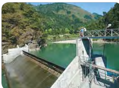
Andhikhola headworks with rubber dam.
