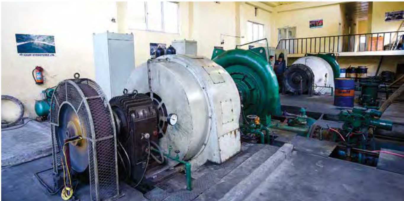
Powerhouse of Khudi Hydropower Project.
