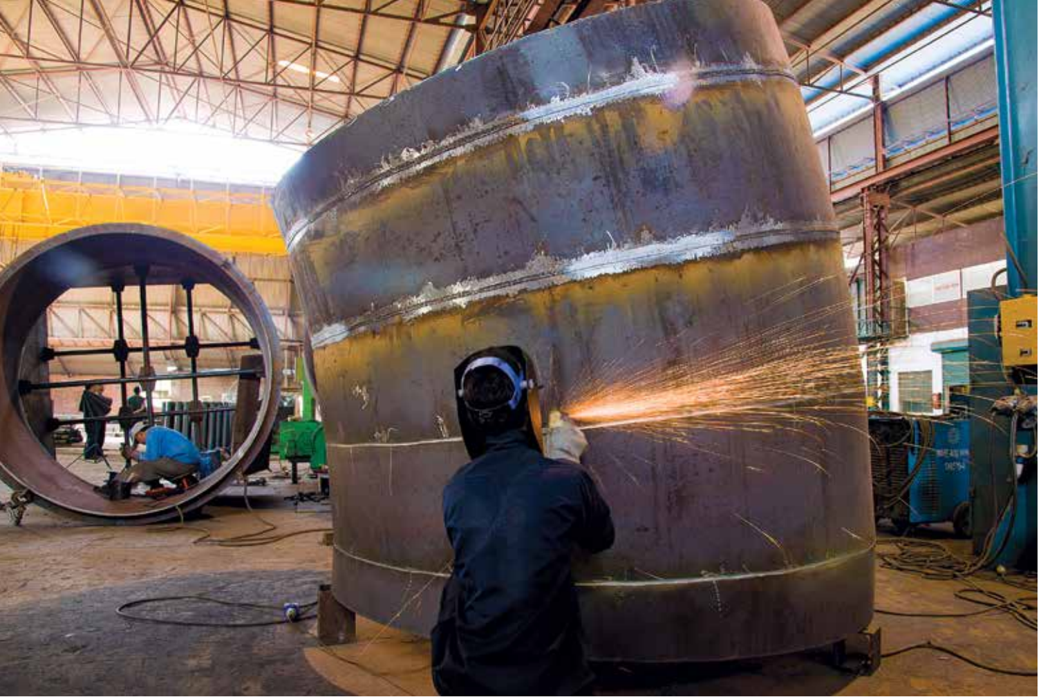
Fabrication works at NHE Workshop, Butwal.
