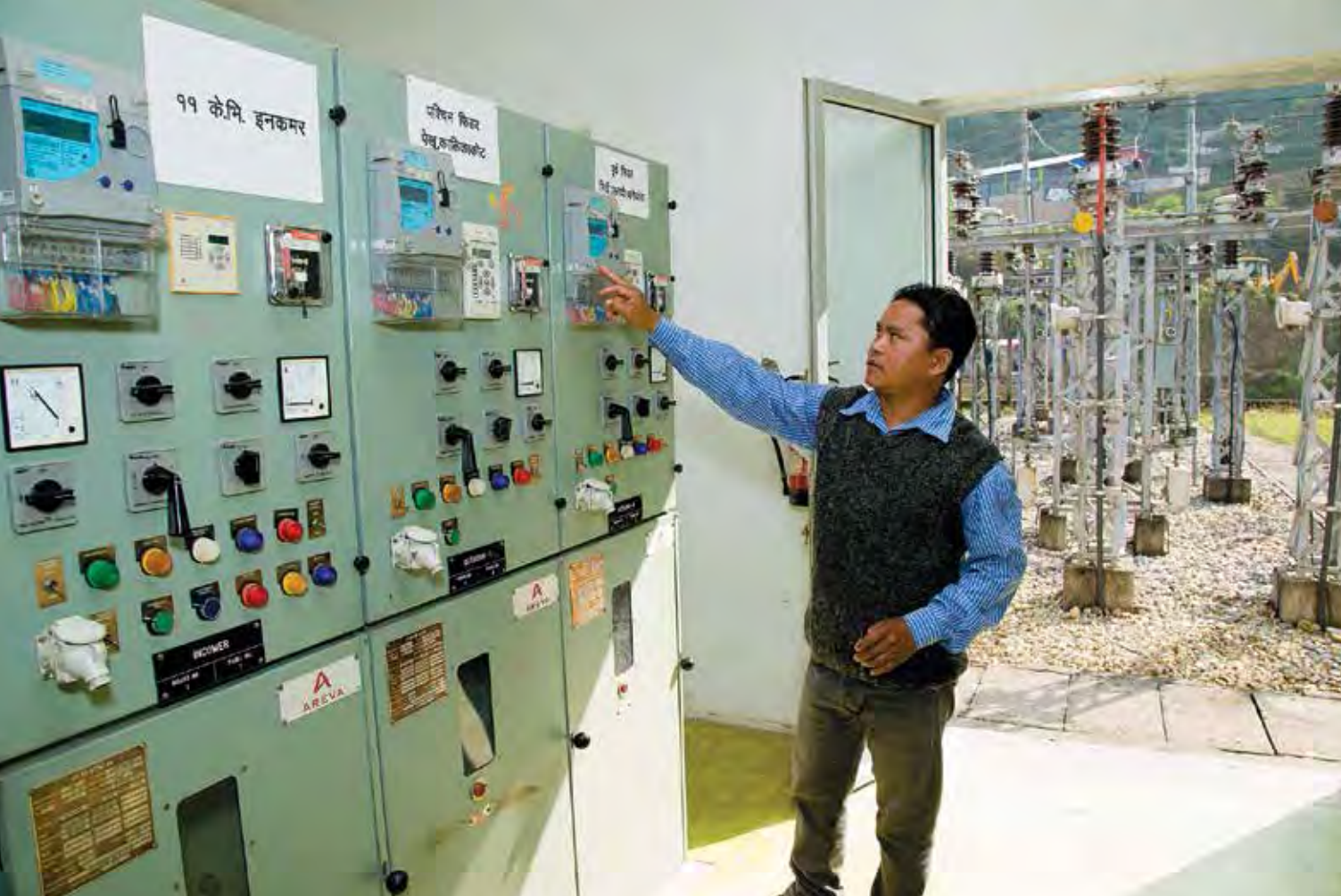
33 KV Mirdi sub-station, Waling.
