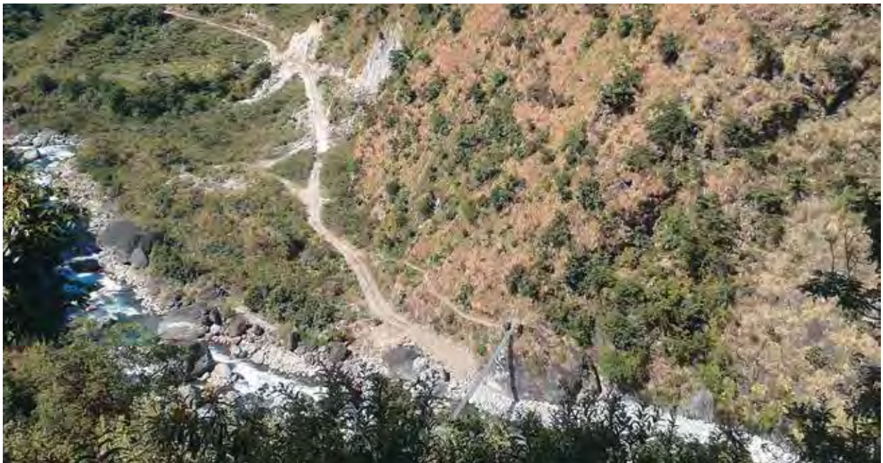
Powerhouse location of 30 MW Nyadi Project.
