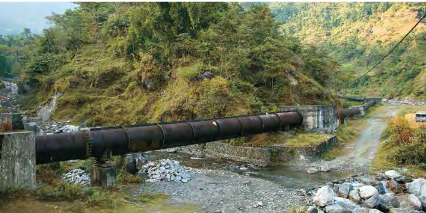
Penstock pipe of Khudi Hydropower Project.
