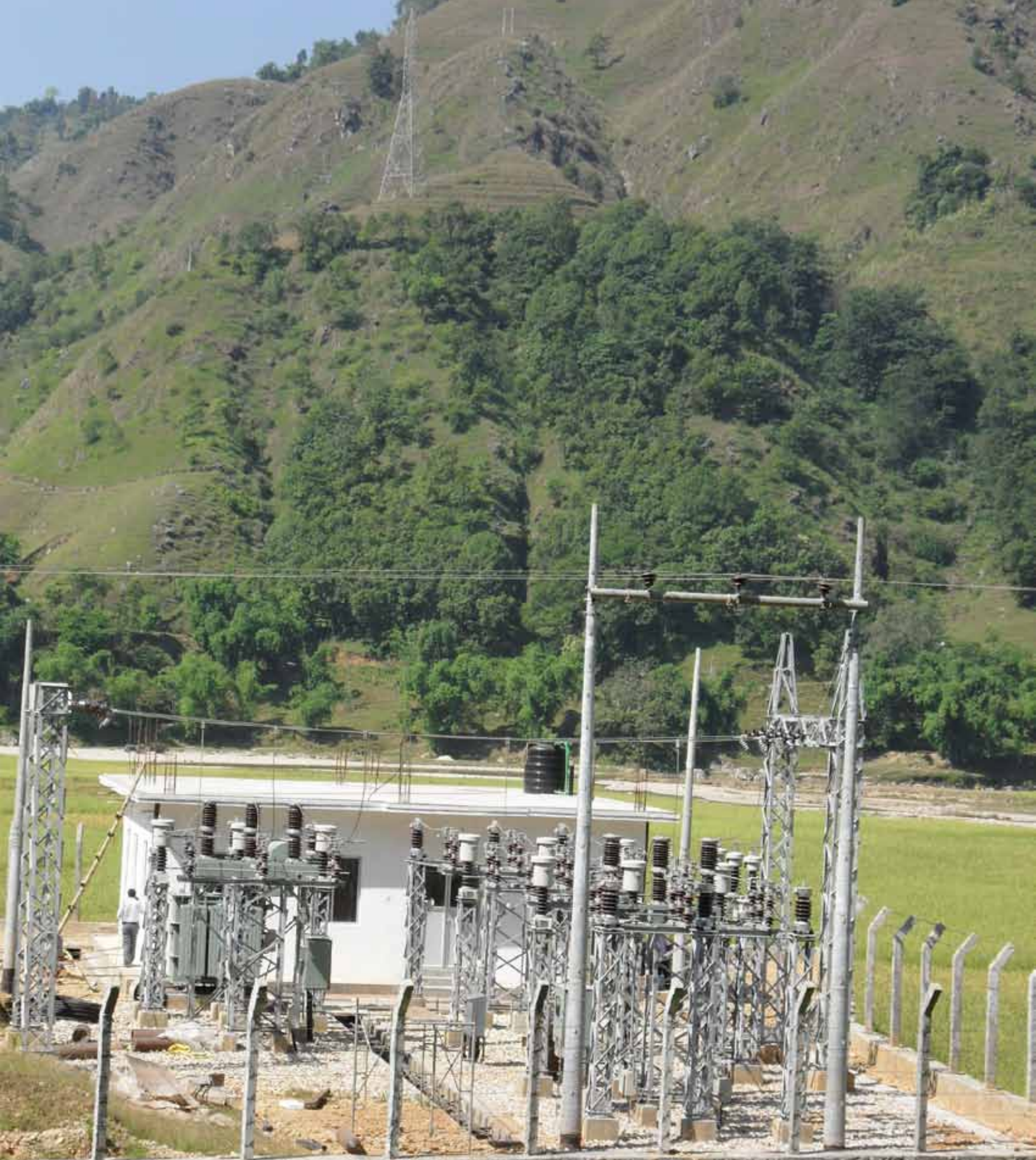
Distribution Sub-station at Mirdi
