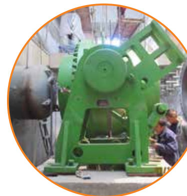
▲ Nyadi powerhouse construction in progress.
