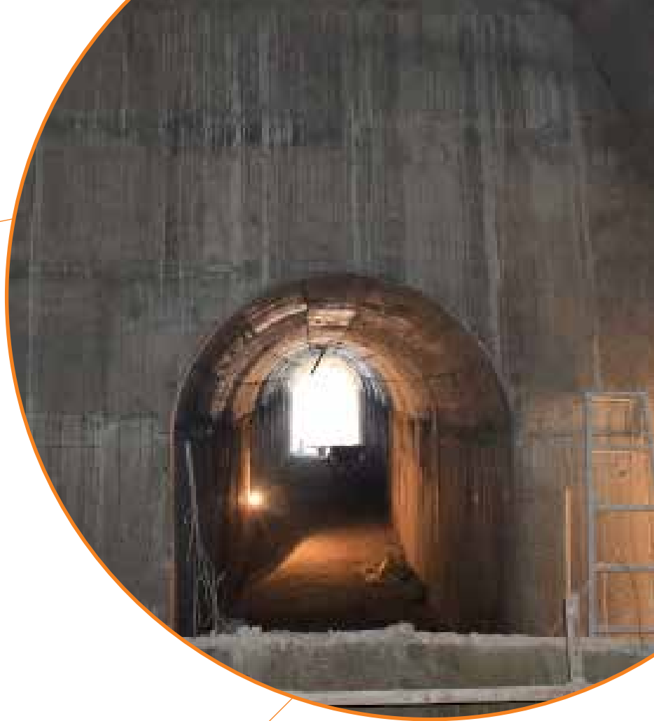
▲ Nyadi headrace tunnel.
