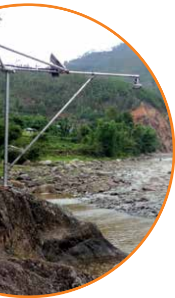
▲ Flood Monitoring System installed in the upstream of Jhimruk Power Plant Dam.
