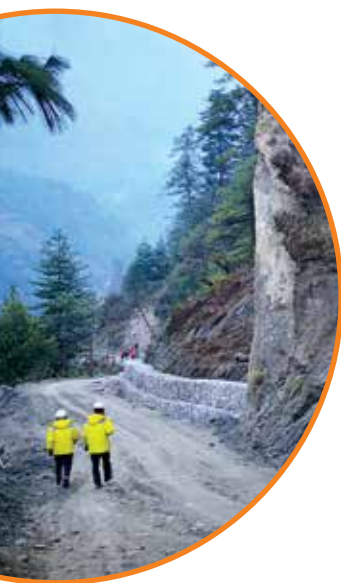
▲ Gabion protection work at Lower Manang access road.
