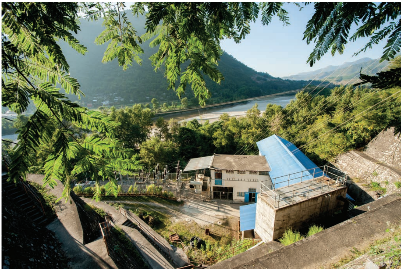
▲ Powerhouse of Jhimruk HEP
