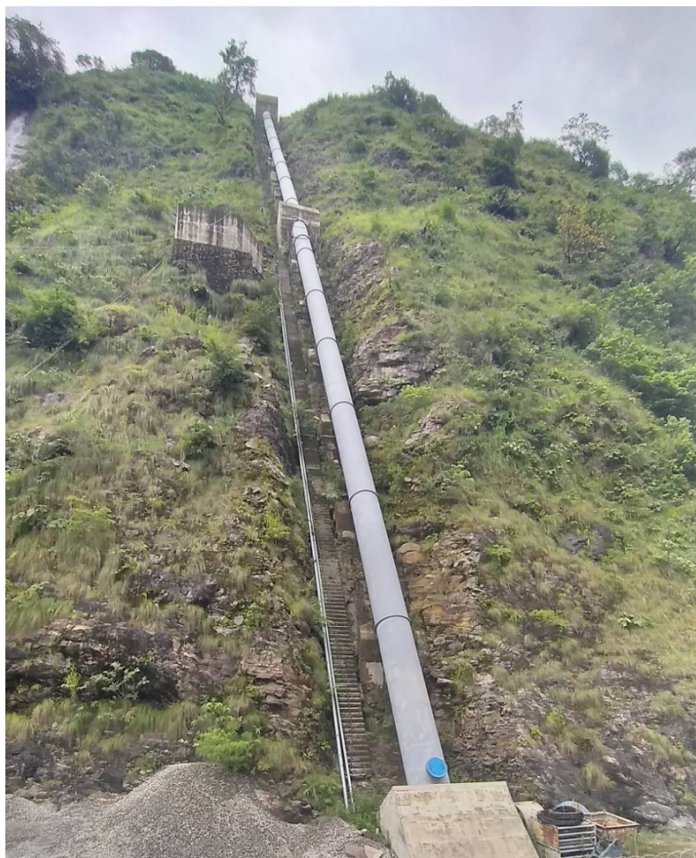
▲ Nyadi Power House
