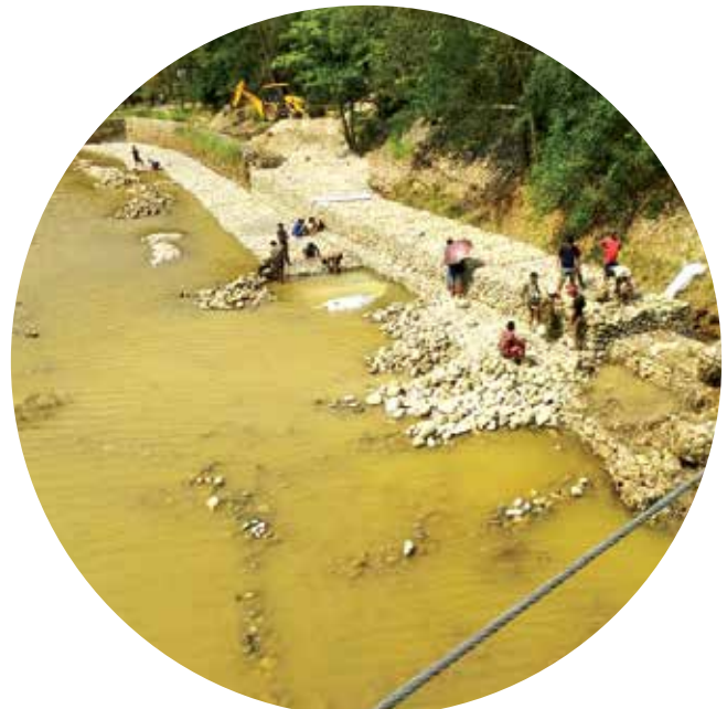
✔ Jhimruk Power Plant: River Training Works
