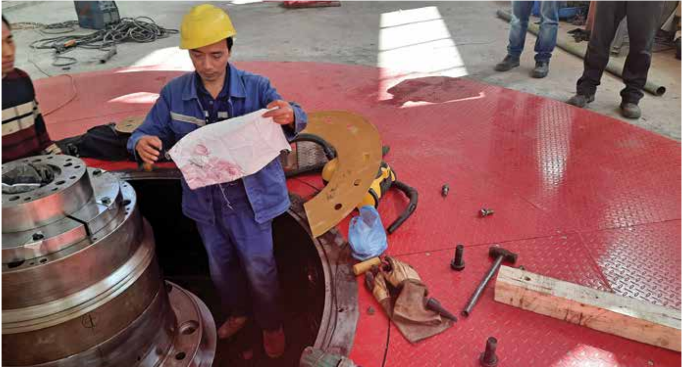
↗ Nyadi Hydropower : Generator installation
