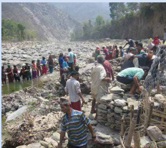
Repairing and maintenance of irrigation canal
