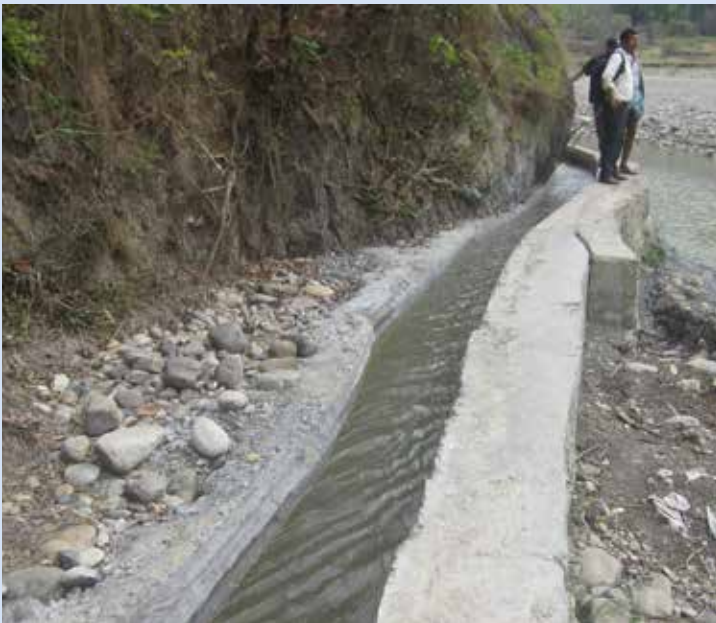
Irrigation Canal Construction
