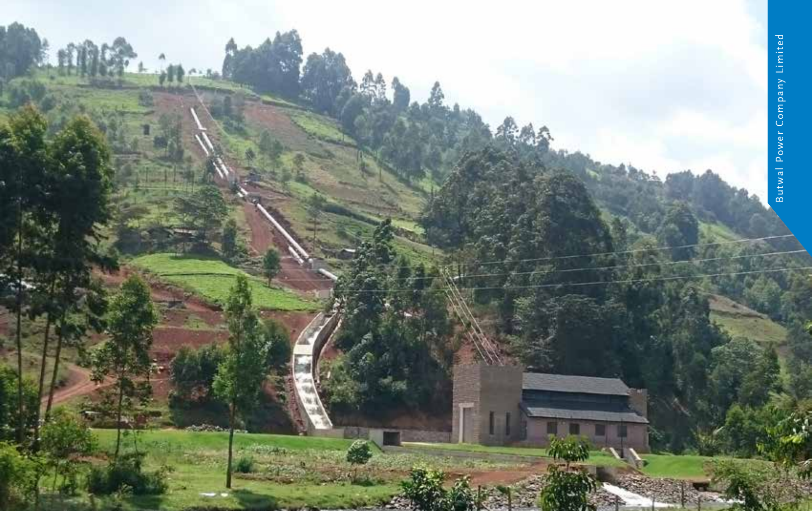
HCE involved in 5.6MW GURA project in Kenya for the project management, design, construction supervision & quality control.
