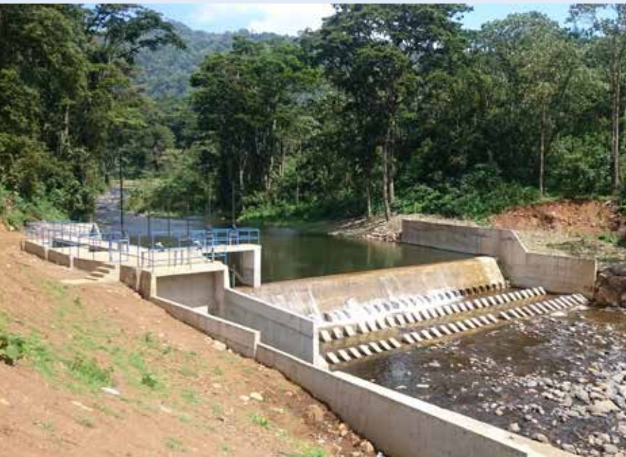
Hedwork site of 5.6MW GURA project in Kenya.
