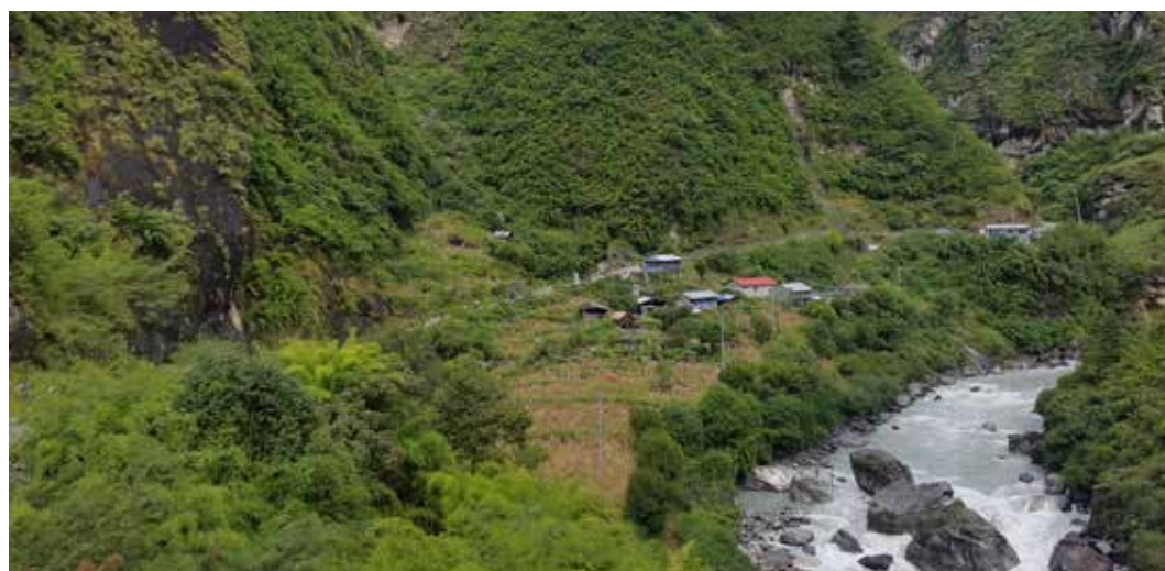
Powerhouse area of Lower Manang Marsyangdi HEP.
