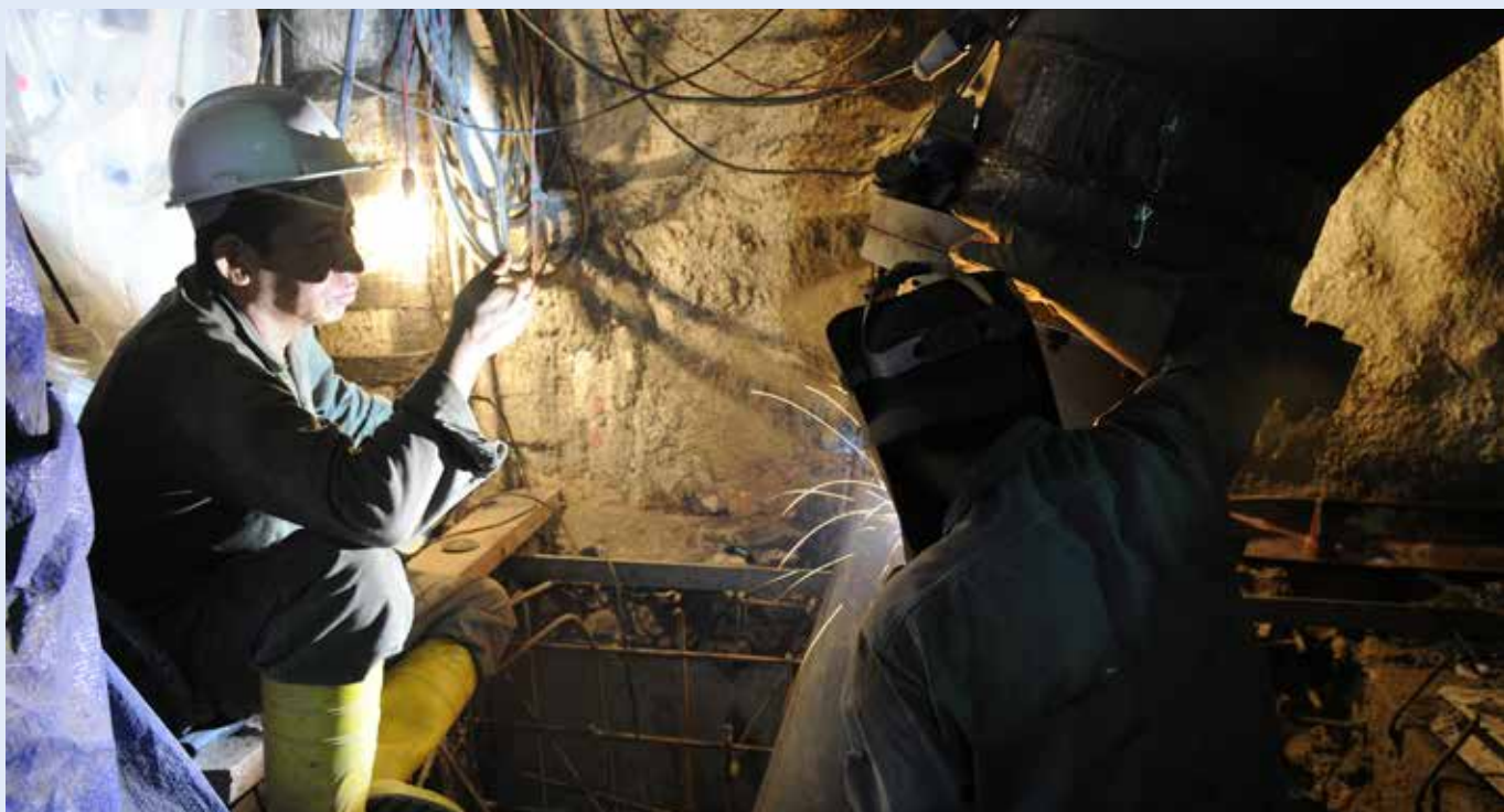
Repair and maintenance work
