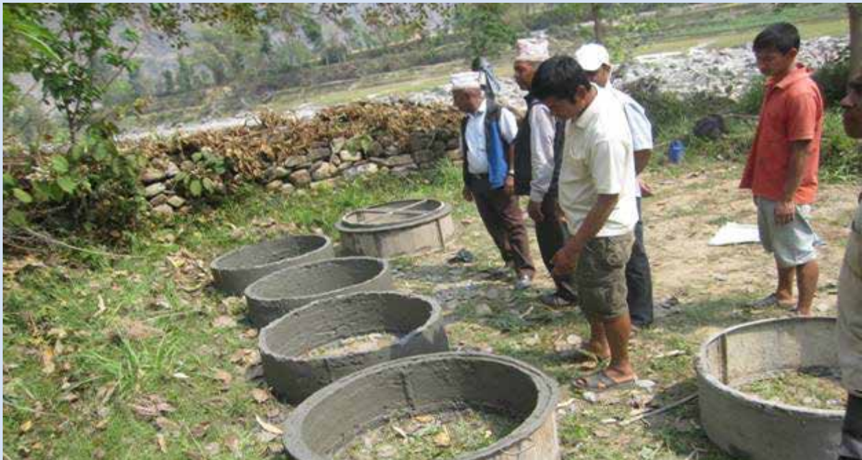
Concrete ring production
