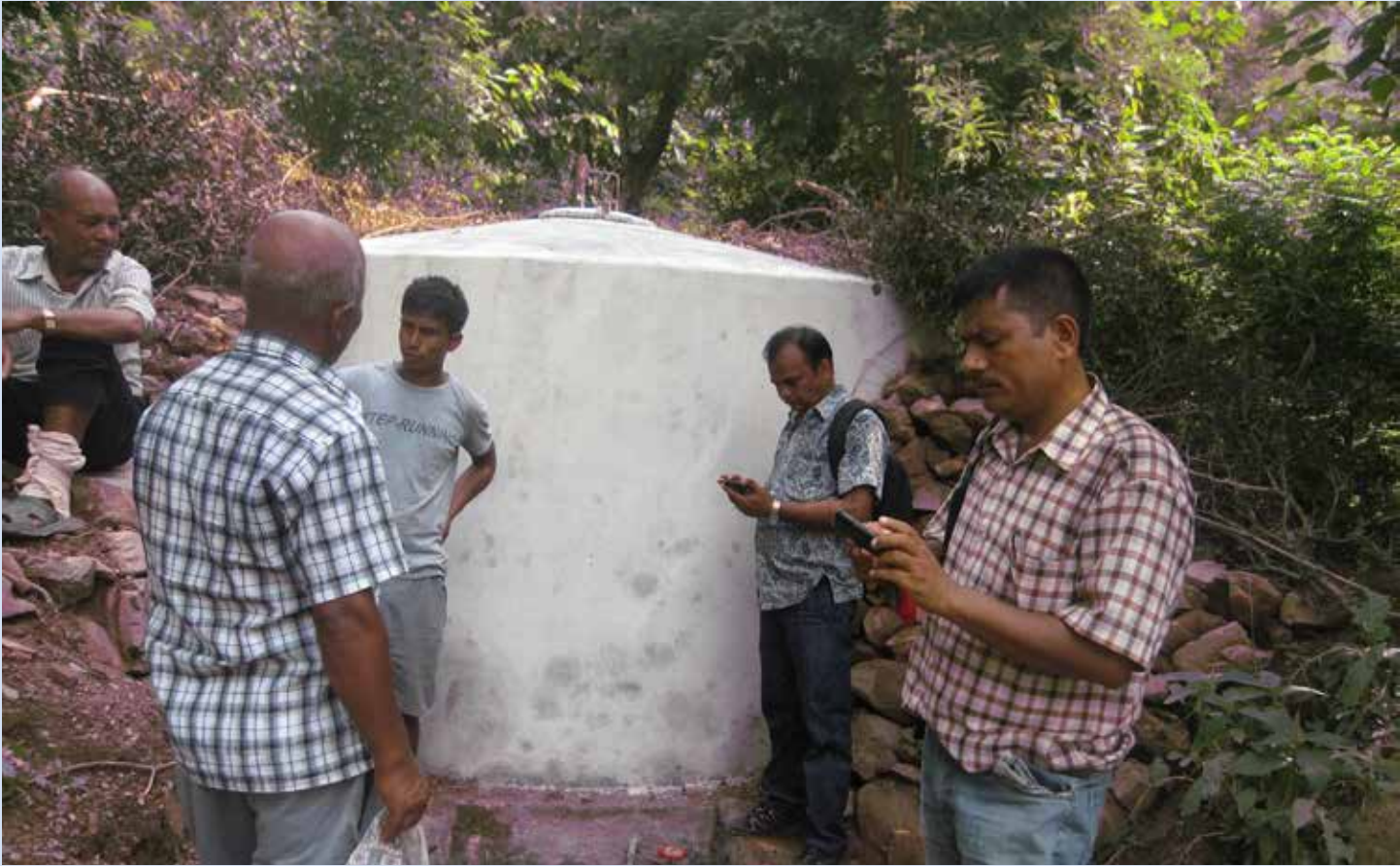
Construction of drinking water reservoir tank
