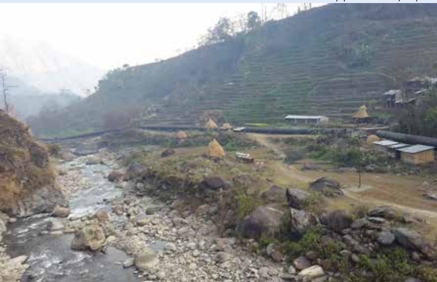
Penstock pipe of Khudi Hydropower
