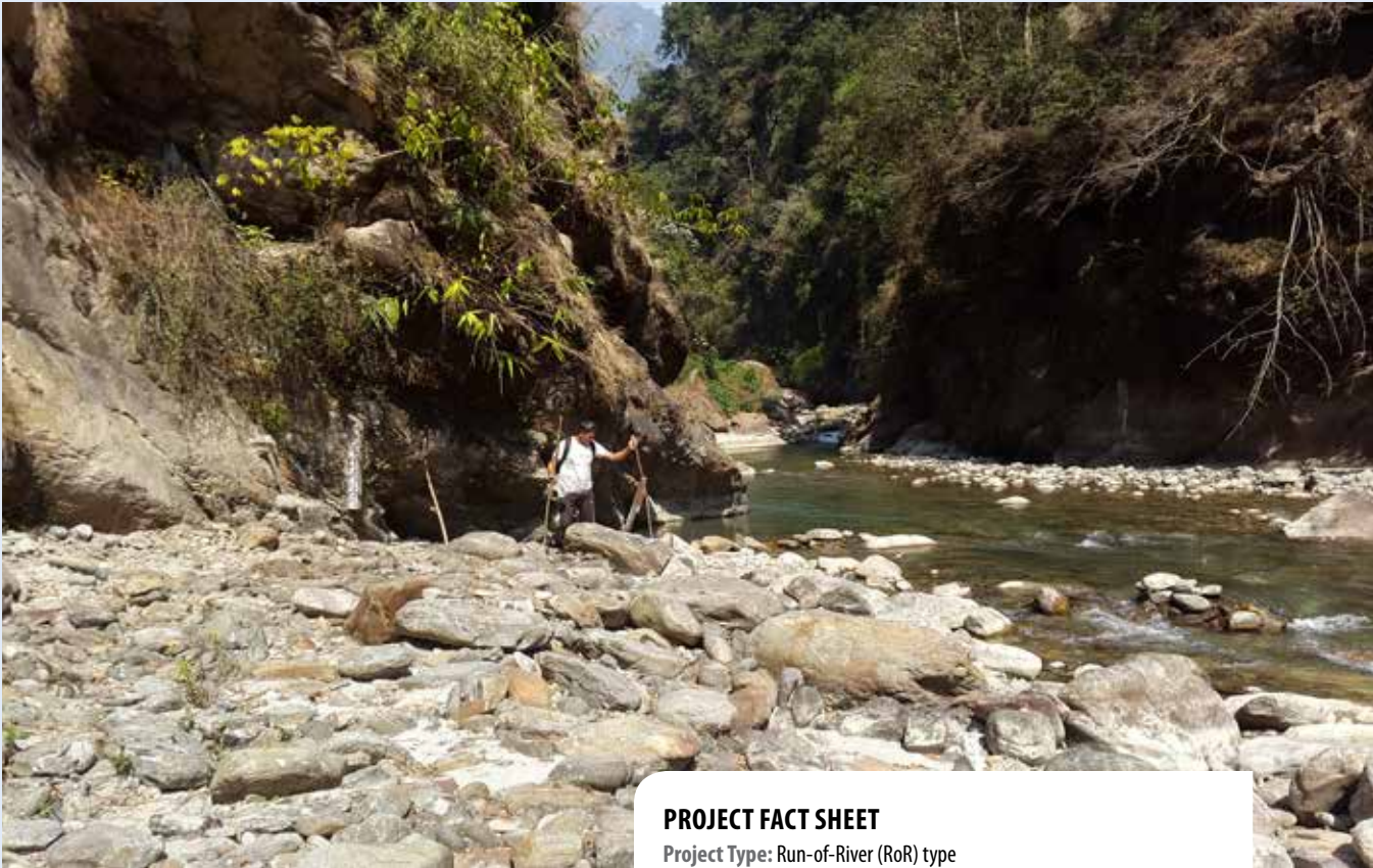
Hedwork site of Nyadi Hydropower
