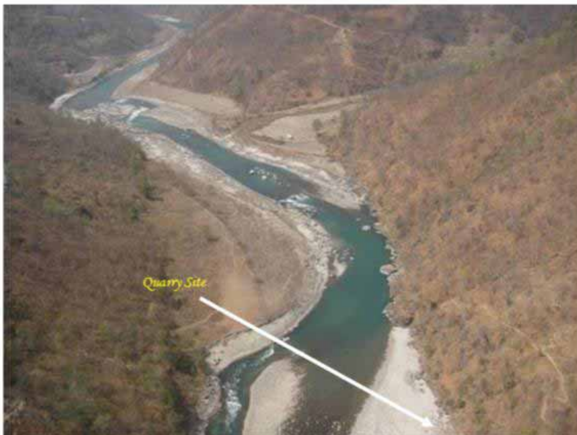
Photograph 2.3 : Location of Quarry Site at Powerhouse
