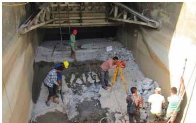
➤ Repair of under sluice-way in Jhimruk hydropower plant.
