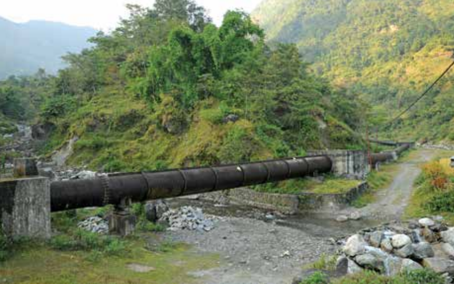
▲ Penstock pipe of Khudi Hydropower Project.
