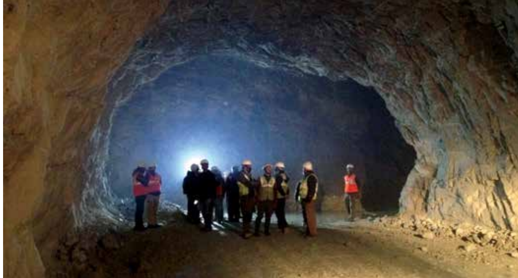
▲ Settling Basin Cavern Mistri Khola Hydropower 43 MW.
