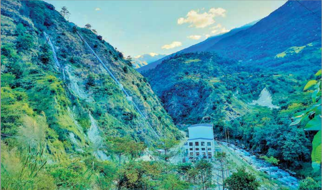
▲ Nyadi HP: Power House and Substation
