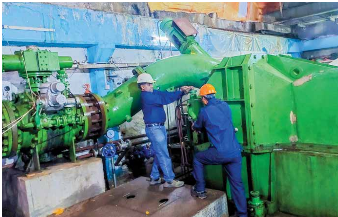
▲ Turbine Maintenance of 9.4 MW Andhikhola Hydropower Plant.
