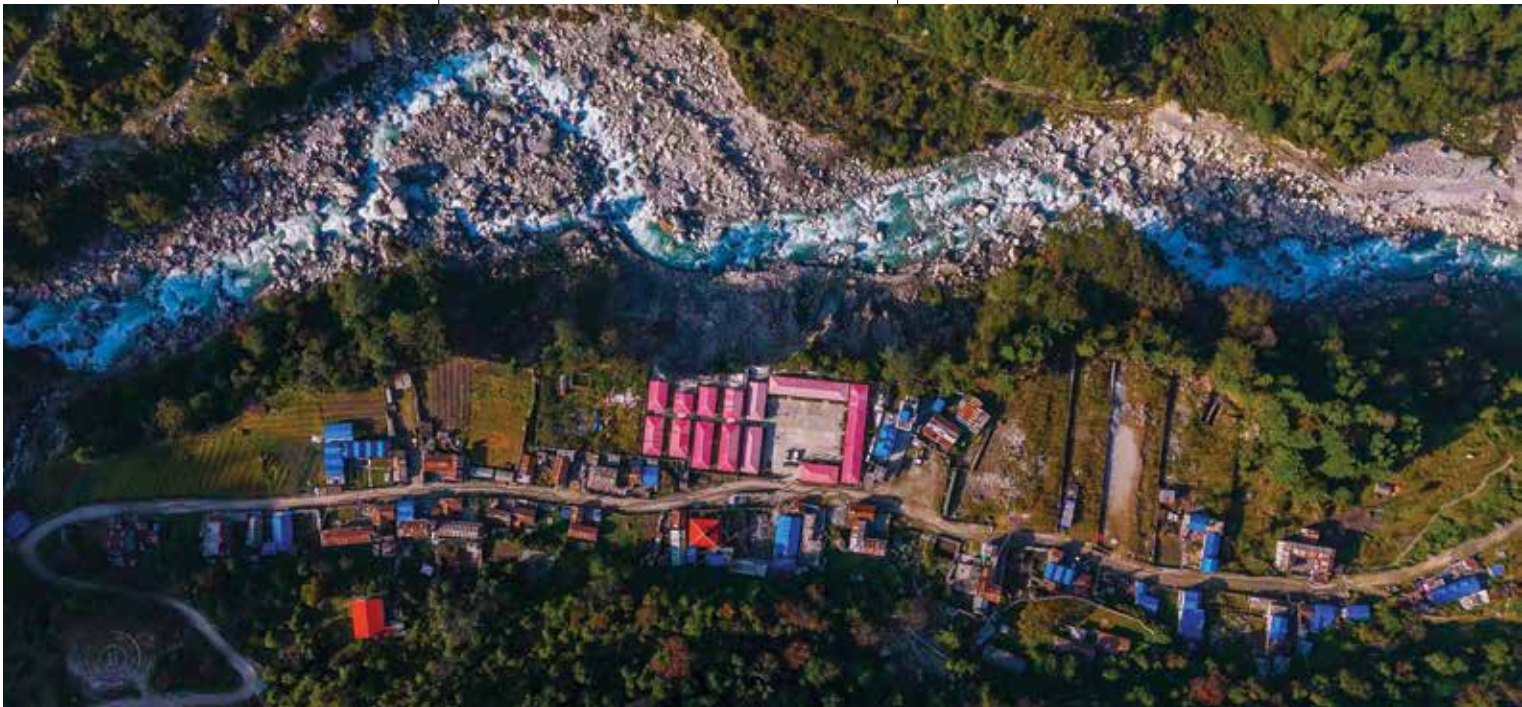
▲ Bird-eye View of Marsyangdi River and MCP Construction Camp
