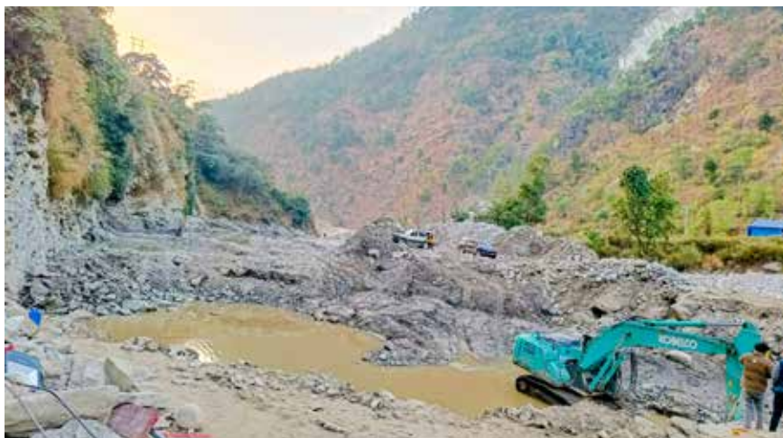
▲ KAHEP: Construction work in progress.
