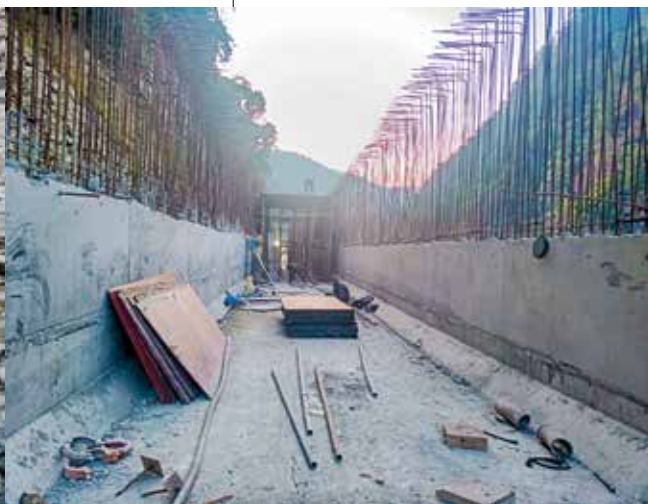
▲ KAHEP: Headrace Canal Construction
