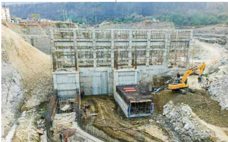
▲ Seti Nadi HPP under Construction Supervision of HCE
