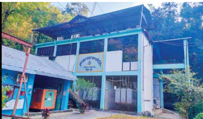
▲ Powerhouse of 9 MW Andhikhola Hydropower Plant.
